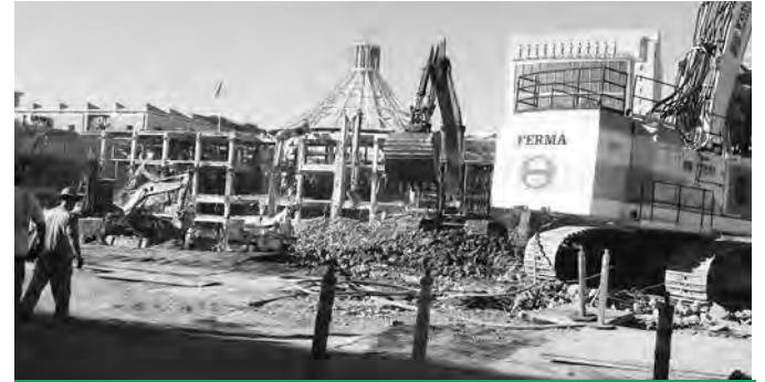
Local 150 members participate in demolishing parts of Sacramento's downtown mall to build the new Golden 1 Center.
